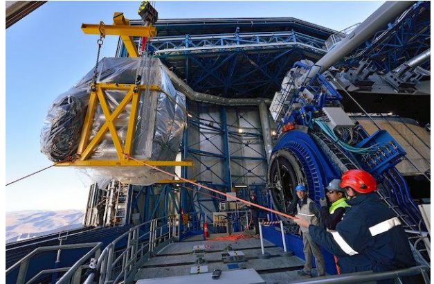
Fig. 3. Installation of MUSE, the Multi Unit Spectral Explorer, on the Nasmyth platform of the 8.2m UT4 telescope of the Paranal Observatory in Chile. MUSE has a total mass of 7 tons.
